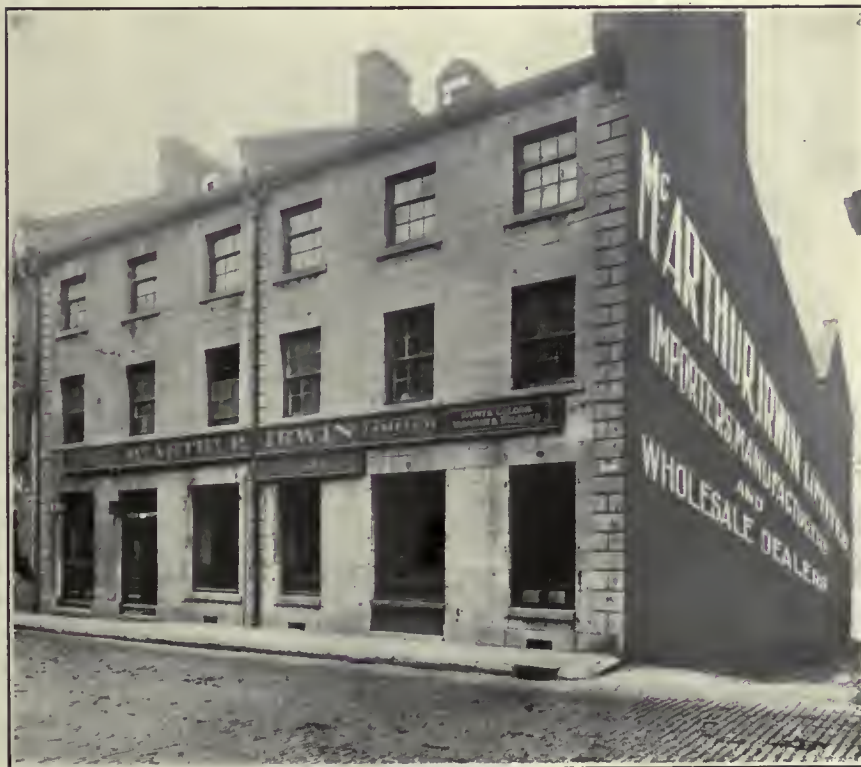
McARTHUR-IRWIN LIMITED. Offices and Storehouse 324 to 328 St. Paul Street.
